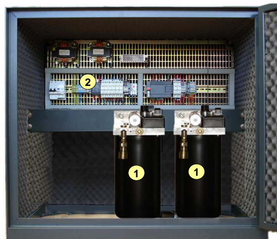
1- Standard hydraulic group, 2- Control panel with AT224 PLC, 1 access, 2 bollards (example)
